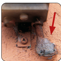
Corrugated pipe entry protection
