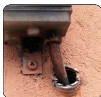
Corrugated pipe entry protection
