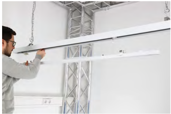
2 - hang new LED modules in old mounting rail
