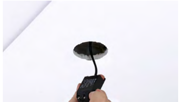
3 - compact power supply unit is inserted into the cavity
