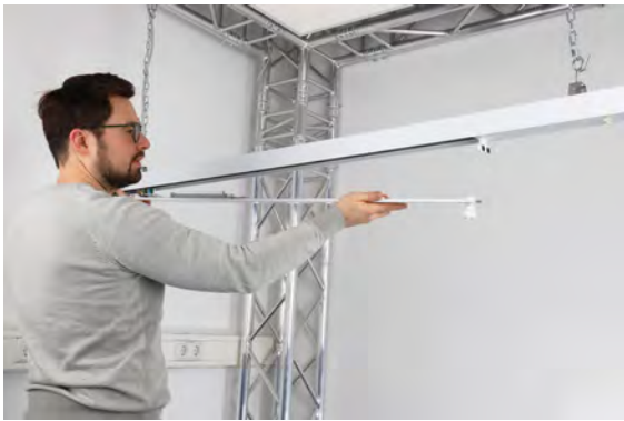
1 - old light inserts removed [wiring remains in]
