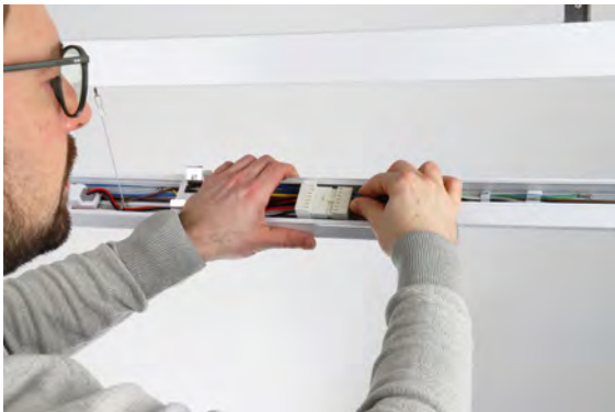
3 - connect modules and adjust power if necessary
