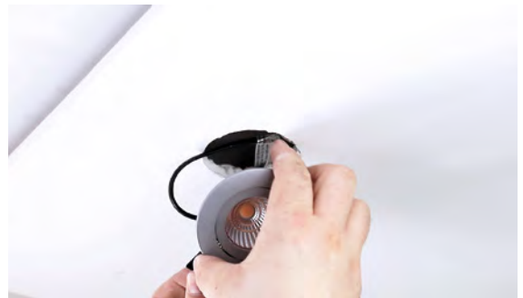
5 - inserting the spot into the ceiling cut-out
